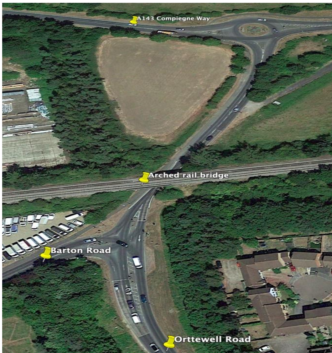
Fig 3 Site of Orttewell Road rail bridge
